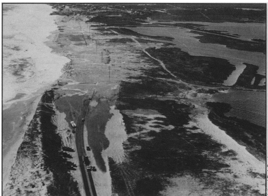
Cape Hatteras after 1973 storm. Overwash destroyed road and built up bayside.
