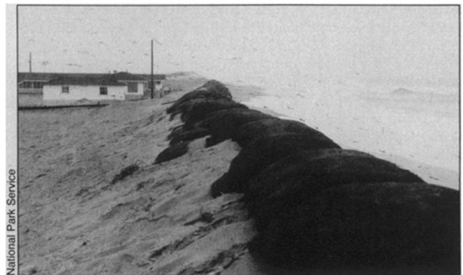
Eight months after $500,000 sand replacement, 700 sandbags, two tons apiece, were placed on this Cape Hatteras beach. Within two months, the bags were destroyed.
