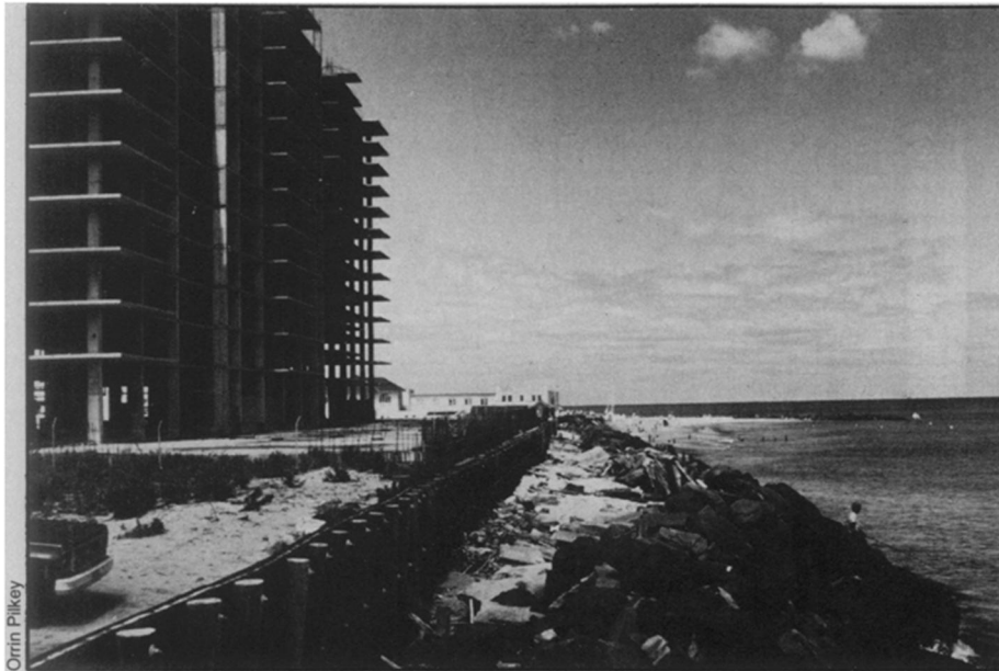
"New Jerseyization" in Monmouth Beach, N.J. Sand has built up around the jetty in the background, while the beach in front of the sea wall no longer exists.
