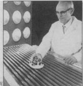
Beneath the cover is a cavity filled with a mat of black fiberglass. Its cylindrical fibers collect and transfer heat to warm air circulating through the cavity — for temperatures in excess of 180°F, if necessary. The system's design also minimizes weight and conductive heat losses with a thermally stable, insulating, foam backing.
