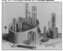
The major piece of equipment pictured is Priestley's pneumatic trough. The scientist used this apparatus to heat substances under water to liberate gases and then to collect those evolving gases in the glass tubes.
