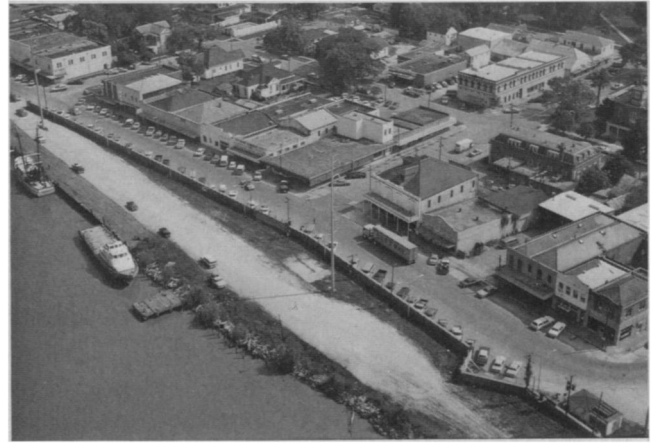
Morgan City, Louisiana, showing flood levees judged "too low" by the Corps of Engineers.
