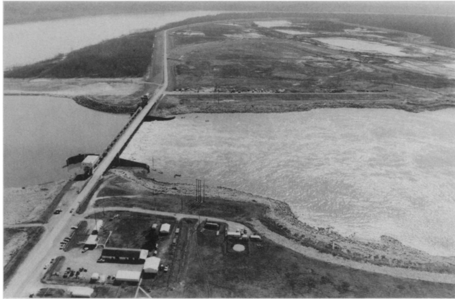
The Mississippi's Old River Control Structure, actually a complex of dams, locks and levees, diverts 70 percent of the river down the main channel.
