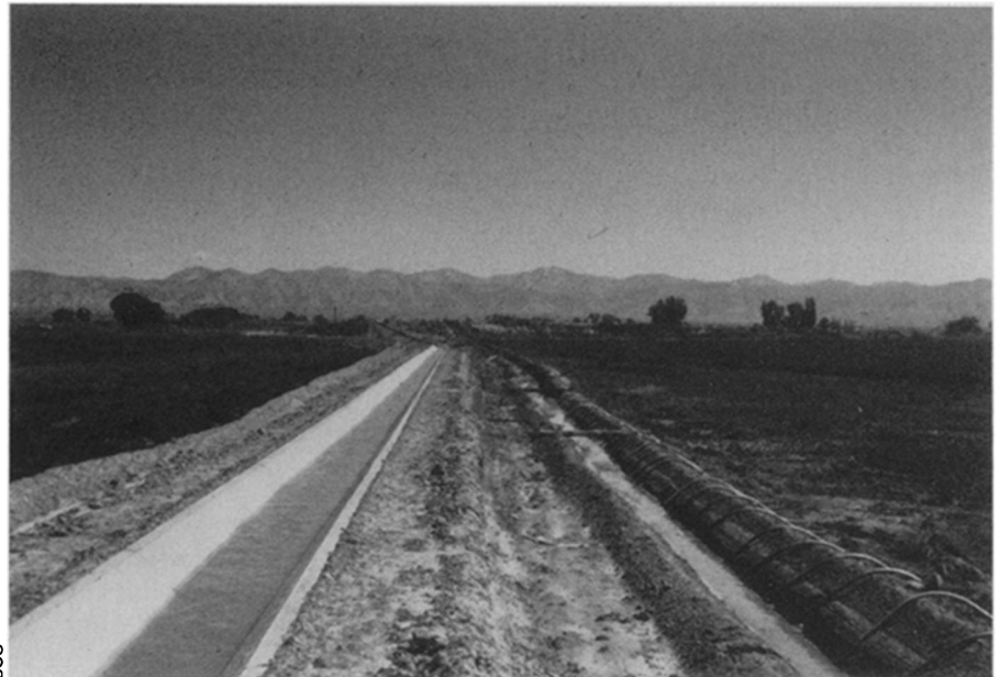
Lining irrigation ditches in cement (left ditch) improves irrigation efficiency by curbing seepage through dirt bottom.
