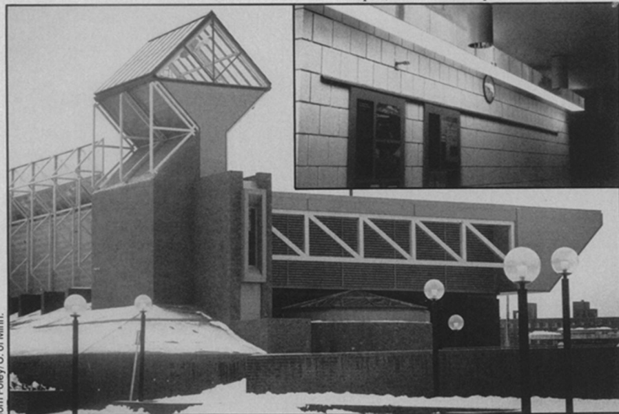
Exterior view of the University of Minnesota's Civil and Mineral Engineering Building. Inset shows a "light pipe" illuminating a hallway.
