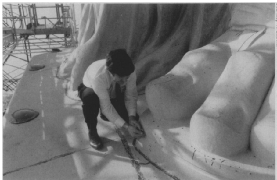
Robert Baboian examines the Statue of Liberty's copper sandal for signs of deterioration. Measurements of the copper skin's thickness provide a benchmark for tracking future corrosion.
