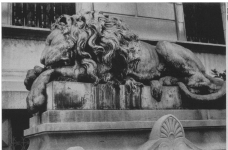
A bronze lion drips corroded metal, staining its masonry resting place.
