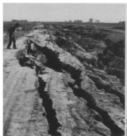
Soil liquefaction during a 1979 Imperial Valley earthquake generated fissures along a canal near El Centro, Calif.
