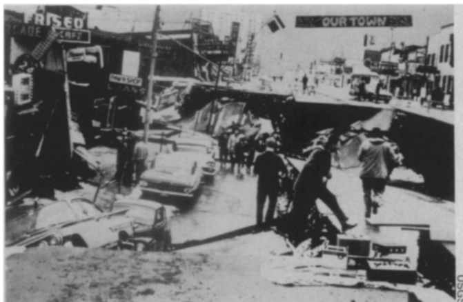
The settling of sandy soil after liquefaction during the 1964 Alaska earthquake caused extensive damage.
