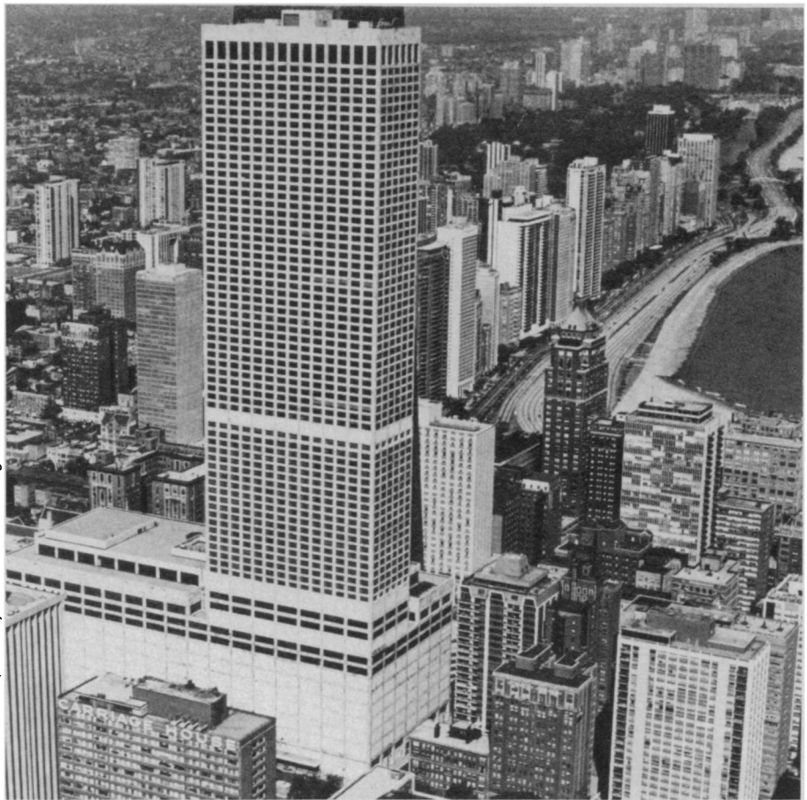
At 859 feet, Water Tower Place in Chicago is the world's tallest all-concrete building. Its construction required special, high-strength concrete.
