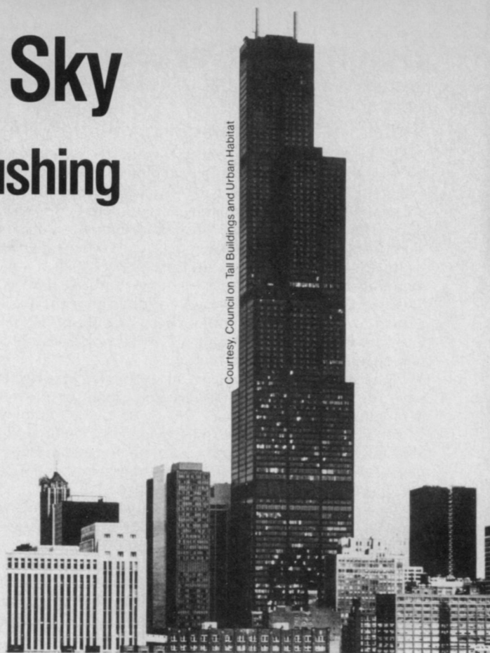
Chicago's Sears Tower, the world's tallest building.
