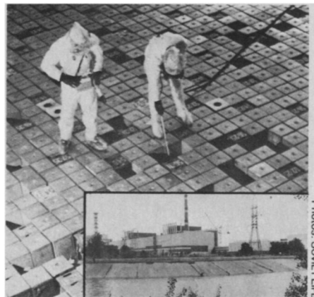
Photo published two months ago shows technicians working on what U.S. experts suggest is probably the Chernobyl reactor core; blocks within grid are probably graphite. Cooling water would circulate through channel holes visible in center of blocks. Inset: Chernobyl plant.
