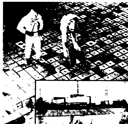
Photo published two months ago shows technicians working on what U.S. experts suggest is probably the Chernobyl reactor core; blocks within grid are probably graphite. Cooling water would circulate through channel holes visible in center of blocks. Inset: Chernobyl plant.
