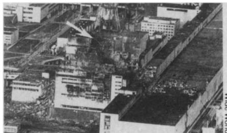
Arrow points to the severe structural damage sustained during an explosion at Chernobyl's #4 reactor.
