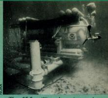
The \$5.5 million Aquarius replaces NOAA's smaller, less sophisticated Hydrolab, which hosted nearly 200 missions before it was retired in 1985. Aquarius, which will get its power and air via an umbilical system connected to a surface support boat, has a sleeping area, showers, laboratory equipment and a galley.
