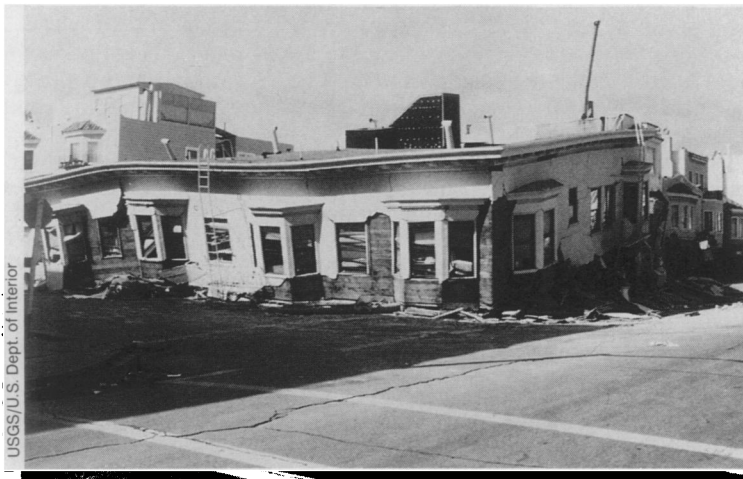
Violent shaking and soil liquefaction in San Francisco's Marina district caused the lower floors of some buildings to collapse completely.
