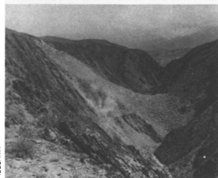
Two photographs show the Uch-Terek valley in Kyrgyzstan before and after an explosively triggered landslide in 1989. The 45-meter-high dam was made to simulate the Kambarata project.
