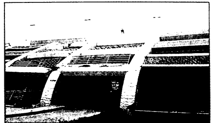
Collapsed parking garage in Northridge.
