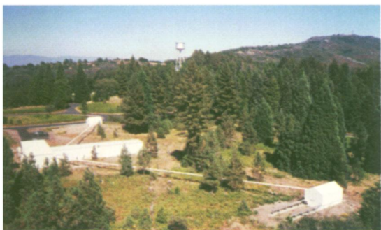
Combining light from two 0.4-meter telescopes located 100 meters apart forms a single infrared interferometer at Mount Palomar Observatory.
