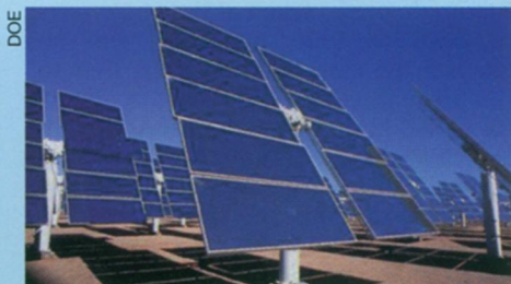
Solar Two's segmented mirrors are mounted on frames that track the sun throughout the day, continuously reflecting light onto the central receiver.
