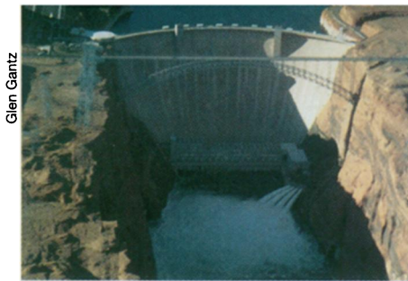
An aerial view of the Glen Canyon Dam on the Colorado River during the flood.
