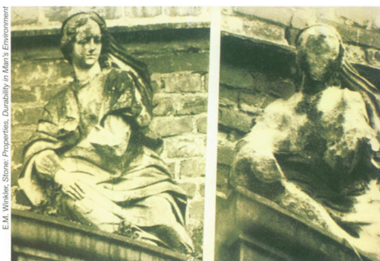
In 1908, a sandstone sculpture on Herten Castle near Recklinghausen, Germany, had eroded only slightly, leaving the features clearly visible (left). By the early 1970s, pollution had chewed away at the sculpture until it was a faceless rock (right). Although the sculpture was carved in 1702, most of its deterioration occurred after industrialization, in the mid-19th century.
