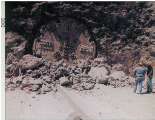
A tunnel-boring machine completed an 8-kilometer-long shaft inside Yucca Mountain in April.
