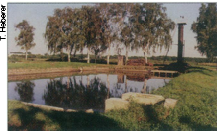
Unlike facilities today, these old-style settlement ponds on a sewage treatment farm south of Berlin rely on light and natural bacteria to cleanse the water. However, drugs and other undegraded contaminants can seep from them into groundwater.
