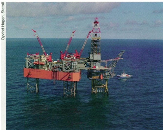
A platform in the North Sea injects liquid carbon dioxide into rocks far below the ocean floor.
