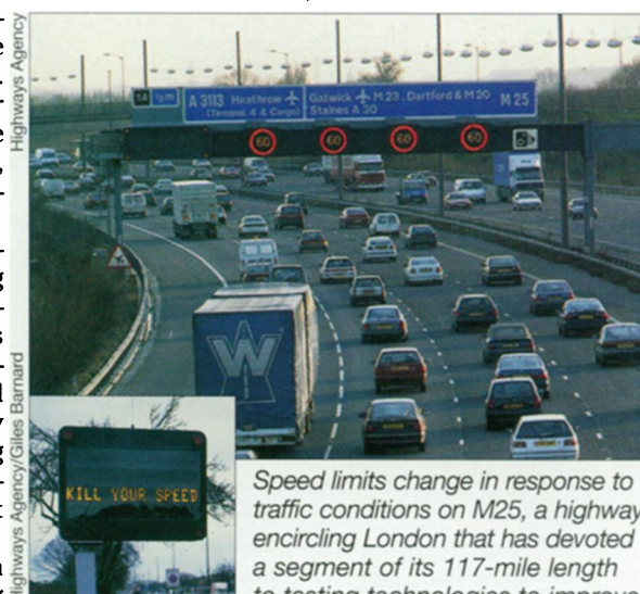
Speed limits change in response to traffic conditions on M25, a highway encircling London that has devoted a segment of its 117-mile length to testing technologies to improve traffic flow. Behind the scenes, people in a control room use video cameras to monitor traffic along M25 and connecting roads. By setting speeds and giving other directions (inset shows a sign on a local road), the pilot system has improved traffic flows, cut accident rates, and lessened pollution, say London police.
