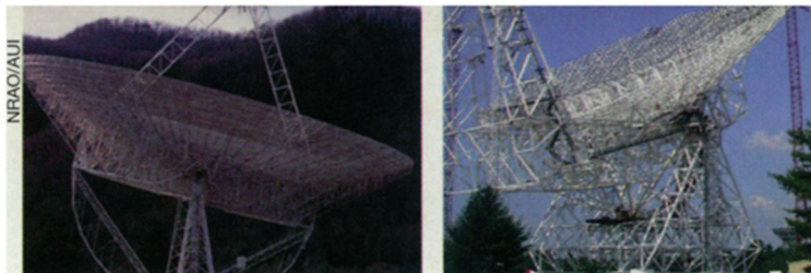
The legs of the tripod supporting the receiver of the 300-foot telescope (left) at Green Bank, W.Va., captured interfering signals. To replace this telescope, which collapsed in 1988, astronomers are building a new telescope (right), whose offset design should minimize interference.
