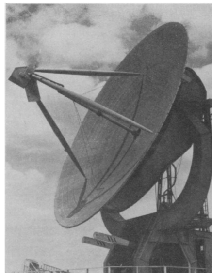
MASER —The solid-state maser shown at the focus of the Naval Research Laboratory's 50-foot radio telescope antenna reflector is being used successfully to detect radiation from Jupiter and Venus. The device is a ten-carat synthetic ruby made to oscillate at microwave frequencies. It increases the range of radio telescopes. (See SNL, May 3, 1958, p. 281 and April 12, 1958, p. 227.)
