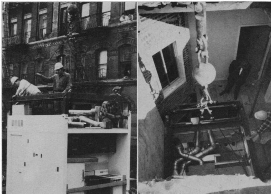
U.S. Department of Housing and Urban Development Pre-assembled kitchen unit provides fast slum rehabilitation (see cover).
