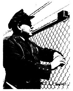
The guard in the picture is reporting "All's Well" to a central guard station in one of our war factories, protected by an acoustic fence. This fence is all ears. If tampered with anywhere, sounds are heard at the central station and an annunciator indicates where the disturbance took place. Even a dog crawling under the fence sets off the alarm. Although the guard in the picture is talking to a detector, he may send a message from any point along the fence by tapping it out in code.
