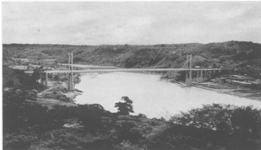
LARGEST LATIN AMERICAN BRIDGE
