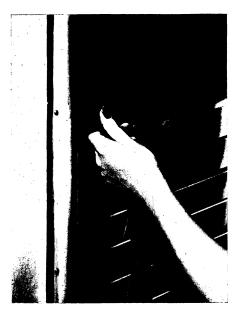
THE PLASTIC STRIP seen on the left side of the picture prevents light from leaking around the edge of a blackout shade. The molding is easily attached to any window frame by means of screws.
