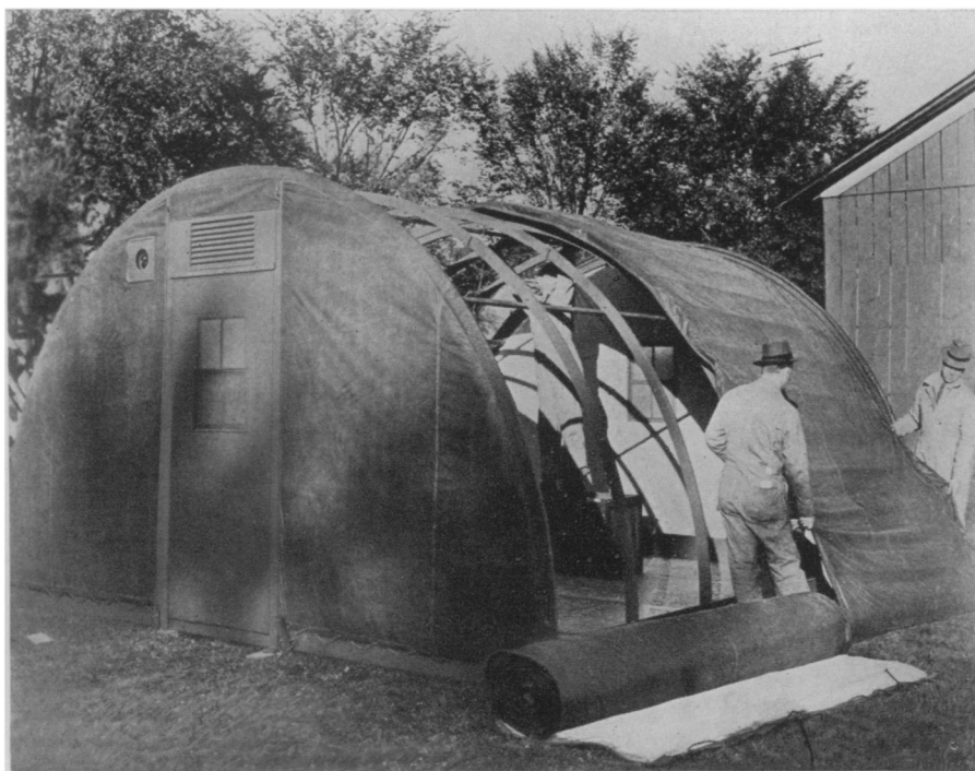
ARCTIC HOME —This portable shelter has been developed for use by Army Corps personnel in cold climates. Blankets of glass fiber insulation in walls and floor save more than 20,000 pounds in the weight of fuel needed to maintain a comfortable living temperature during the heating season. The shelters are lightweight and compact for transportation by plane.
