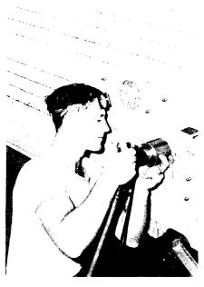
A MAGNETIC RIVETING device, shown in the photograph, speeds certain riveting operations in warplane construction. The device magnetizes a bucking bar which is pulled through narrow channels by a wire, permitting a new type of assembly impossible under old riveting methods in which a bucker, teaming up with the riveter, holds a bar in place manually.
