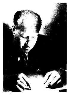
FLUORESCENT — This new fluorescent material illuminates the face of the discoverer, Dr. W. A. Weyl, of the American Optical Company and Pennsylvania State College, with a warm yellow light when it is exposed to ultraviolet light from the lamp at the right.
