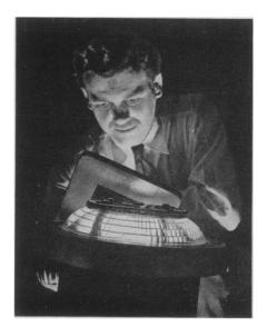
planes. The guiding light continues to burn under a 50-ton load, nearly three times the strength of former lights. Designed in about the size and shape of a fire hydrant, the unit is buried underground except for the top three inches.
