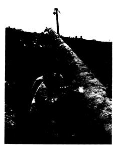
BIG INCH—When this oil line, reported to be one of the largest ever built, is completed, it will have a capacity of 300,000 barrels per day. This photograph from the Lincoln Electric Company shows some of the welding that made it possible to rush it through in record time.
