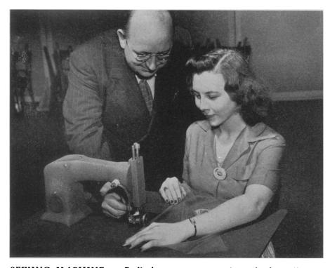
SEWING MACHINE — Radio-frequency current instead of needle and thread is used by this "sewing" machine to join plastic materials. Dr. George H. Brown, RCA scientist under whose direction the electronic machine was developed, shows a worker how to "stitch" a thermoplastic fabric. Although still in the development stage, the machine has possible applications to war production as well as postwar uses.
