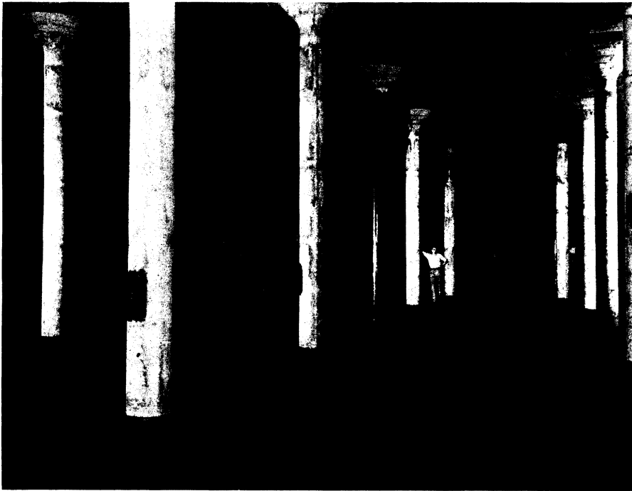
GASOLINE BOMB SHELTER —This is an “inside” view of one of the vast concrete tanks now being built far underground at strategic coastal points and naval outposts to protect from bomb damage millions of gallons of aviation gasoline and diesel fuels. Everything in the tank is lined with synthetic rubber sheets.
