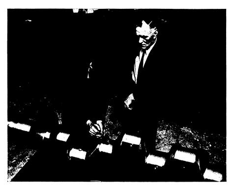
SOLUTION—Dynamite is the new answer to the problem of how to remove a drill broken off in a crankshaft. In this method, devised by Nels Sorenson, right, of the Ohio Crankshaft Co., a small amount—less than a thimbleful—of dynamite is pushed into the hole and set off with a fuse. The pressure of the blast is said to follow the drill flutes to the bottom of the hole, there reversing itself to drive the drill free. A plank laid over the hole stops the drill as it flies out.
