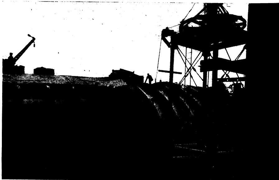
FIRST OF ITS KIND —This is the NACA's new and unique altitude wind tunnel under construction at the Cleveland Airport. The tunnel is insulated by fiber glass.
