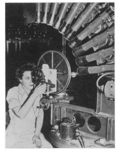
TUBES in the radially mounted battery of collimators shown in the picture contain tiny illuminated cross threads, somewhat like those in a telescope, which look like distant stars seen by a navigator using a sextant. These "indoor heavens" are used to calibrate and test aircraft sextants before delivery to the armed
