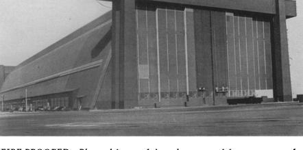
FIRE-PROOFED—Plywood is now being given a special treatment so that buildings, such as blimp hangars, can be made of wood without danger of fire. The wood is impregnated under vacuum pressure in heavy steel cylinders, so that the wood cells throughout the plies are filled with a flame-proofing combination of phosphate, sulphate and boron. The picture shows workmen applying camouflage paint to the plywood-pannelled doors of a West Coast
