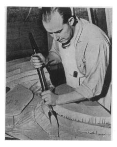
quickly by this means than with ordinary hand chisels. The picture shows one in use.
