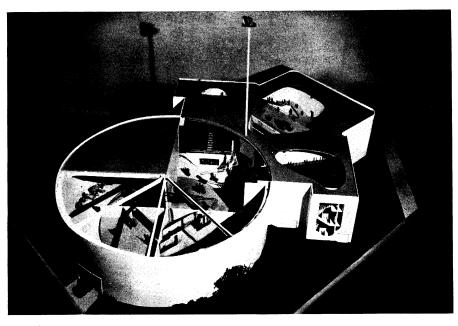
FOR THE FUTURE—A revolving stage will make it possible for two audiences to watch by turns or simultaneously the television broadcasts of the post-war world in a studio built after this model. A single set of controls, cameras and broadcasting equipment will be adequate to handle continuous network schedules without interruption for changes of scene or studio audience.
