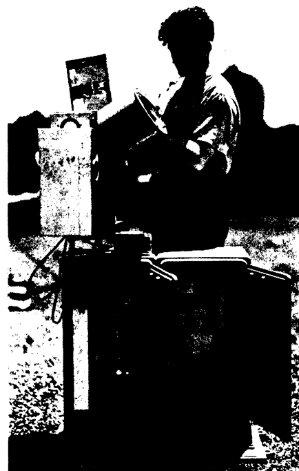
CHECKS CEILING — Airplane pilots can have continuous information about the height of the clouds by means of this instrument, the ceilometer, shown here with Laurence W. Foskett, of the U. S. Weather Bureau, one of the inventors.
