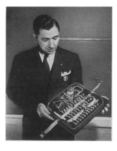
weight, safe, and permit inspection without opening. Flat plates, either plastic or metal, are used as bases for the attachment of all wiring. A typical box is shown in the picture.
