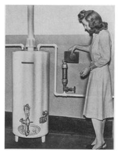
CHEMICAL solution feeder, shown in the picture, permits the housewife to insert into the plumbing system compounds to remove scales and corrosion from the inside of pipes, tanks and boilers. Several chemical compounds for this purpose are available, one being a soluble sodium-phosphate glass.
