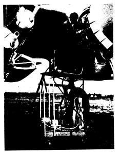
PORTABLE PRE-OILER—This compact device delivers pre-heated oil under pressure to the engines of B-26 Marauders. Developed at the Glenn L. Martin Company, it has demontrated its value both as a saver of man hours and a preventer of failures due to improper lubrication of an engine prior to its first start.
