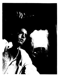
ARTIFICIAL CLOUDS—Created in a bottle from liquid air and warm water, they are used to test insulating materials for the electrical systems of new bombing planes at the Westinghouse Research Laboratories.
