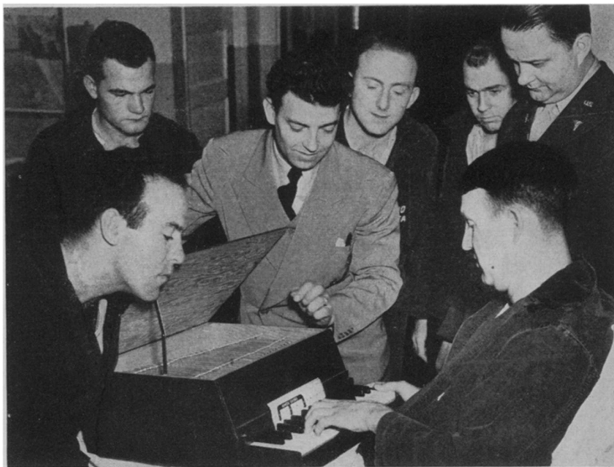
LAP-SIZE PIANO —Harold B. Rhodes demonstrates his new portable piano, which he invented for bed-patients, to soldier patients at Bolling Field Hospital. In building this instrument with filed tubes instead of strings, he used aluminum tubing from the hydraulic system of wrecked planes and plywood from abandoned engine crates. Eight models have already been built for demonstration at each of the AAF convalescent hospitals in this country.
