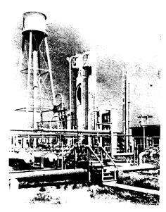
HELIUM EXTRACTION—This imposing array of pipes and towers at the carbon dioxide removal plant represents an important phase at the Bureau of Mines helium plant at Exell, Texas. The plant is the point of origin for a new 2-inch line which permits direct pipe line transportation of helium to the Bureau's Amarillo, Texas, extraction plant or to the Cliffside natural gas field where an underground helium "warehouse" has been established. (See SNL Mar. 17.)
